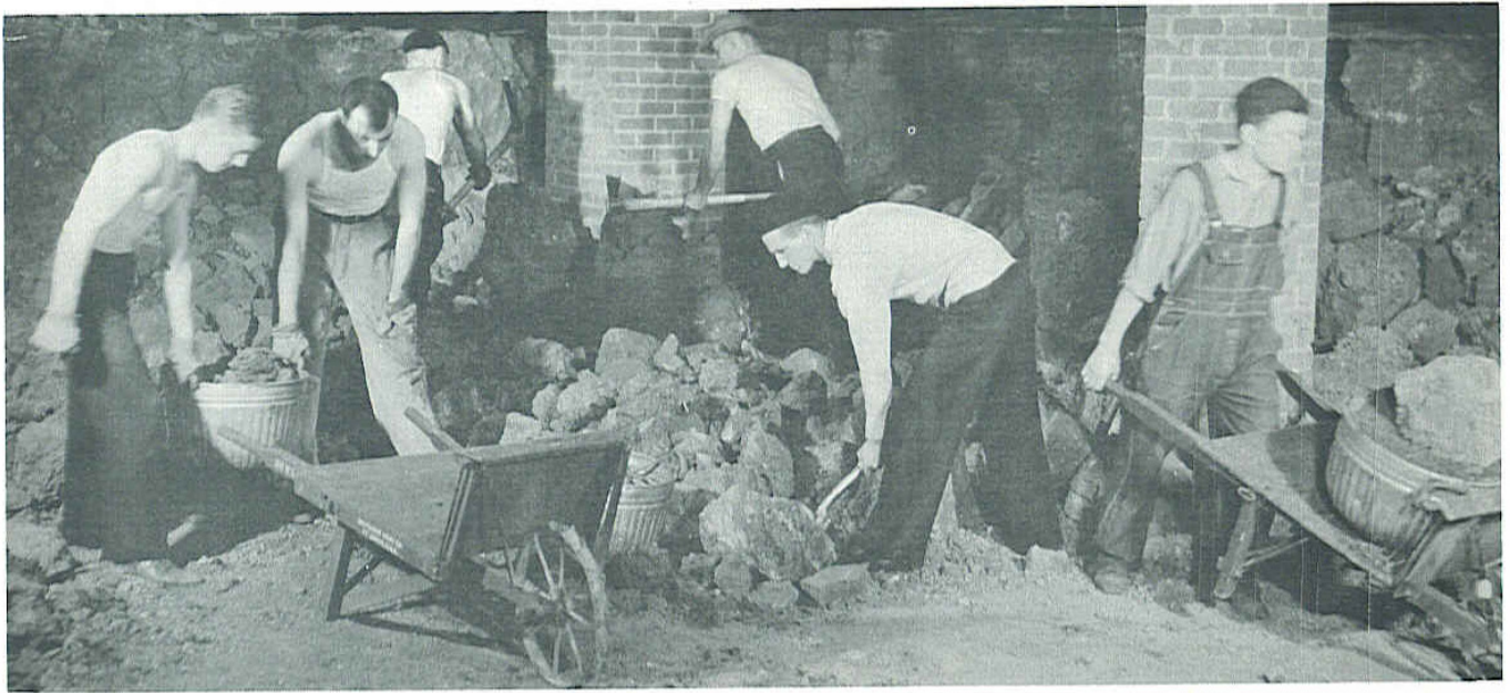
Students excavating for enlarging and new rooms in the basement
